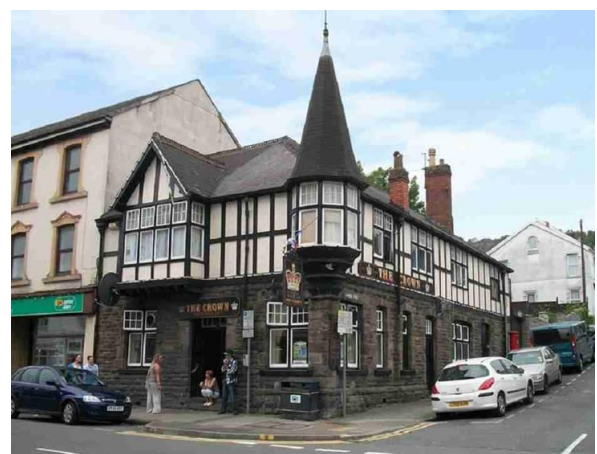
The Crown Inn Morrison, now vacant
